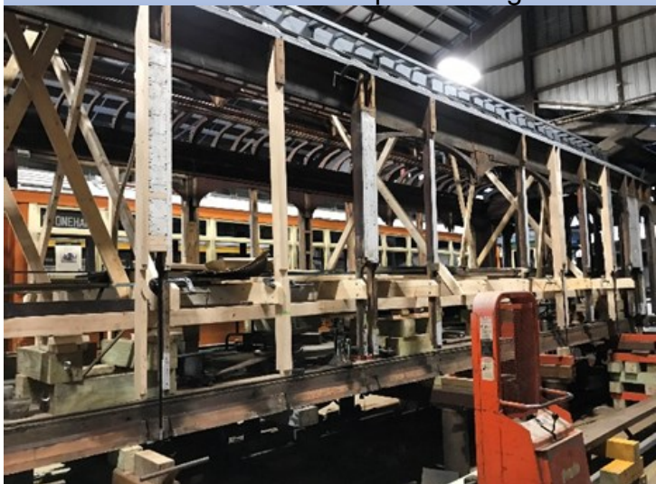
The Narcissus with the new posts being installed.
